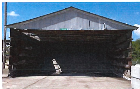
Gage – Under Construction
