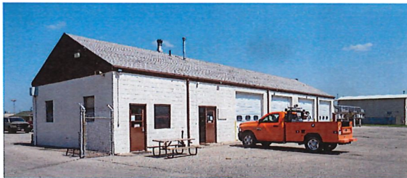
Clay Center Before
